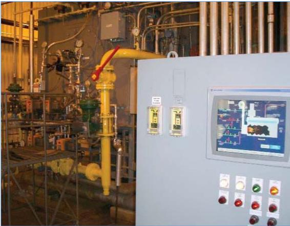
The controls associated with fuel flow and combustion air flow need to be engineered to cope with the variable heat content of LFG. The complexity of the burner management system will depend upon whether the boiler is to be co-fired with natural gas or oil and whether the boiler is to be co-fired at all times or if there will be times when it will be fired with LFG only. Today's modern controls,
