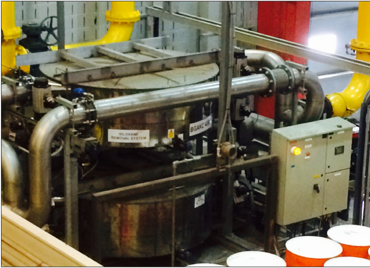
Pictured is a biogas conditioning system at a waste water treatment facility. Venture was contracted to perform a study evaluating a CHP system to generate hot water for heating and process use, and electrical power for the plant use. The biogas system is used to fuel reciprocating engine generators.
